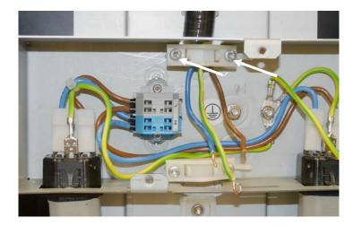
Install the cables as shown in the picture below. If it is a flexible wire, listed as ring pressure-terminal connectors recognized for the wire size must be used. The bonding conductor shall be routed so as not to be exposed to physical damage.
