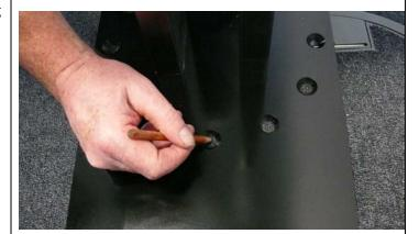
2. Slide all necessary cables (power cable, LAN cable, etc.) through the opening in the base plate positioned above the floor cable outlet.
